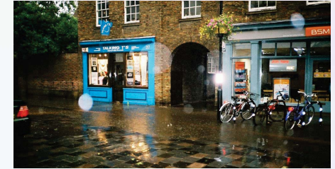
Local flooding due to a storm sewer blocked with leaves in Cambridge, UK (Ilan Kelman).
