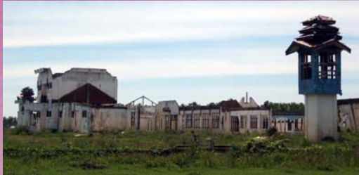
Tsunami-destroyed prison in Aceh (JC Gaillard).
