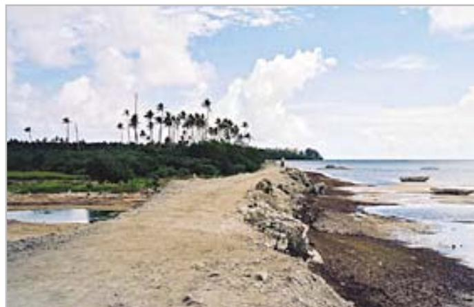
A seawall in Tonga Islands damaged from wave force impact. (Photo source: I. Kelman)
