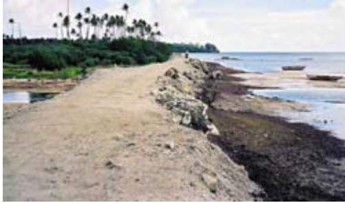
New structural sea defences for low-lying Tonga: a sustainable disaster-risk reduction, or a stopgap measure until a major event destroys them?
