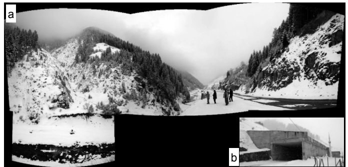
Fig. 3. (a) An avalanche track in front of the road D925 going to Ovit pass, not far from the Sivrikaya settlement, Rize province, Turkey. Road is placed at an altitude ~30 m higher than the bottom of the valley; even though the rock wall next to the road can be reached by an avalanche - some trees over it have lots of broken branches; (b) Avalanche tunnel, Sivrikaya settlement.
